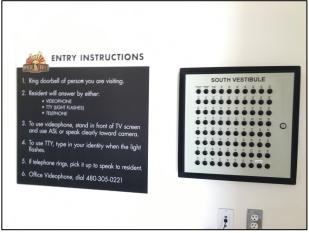
Apartment Light Notification System for Door, Fire Alarm and Phone
